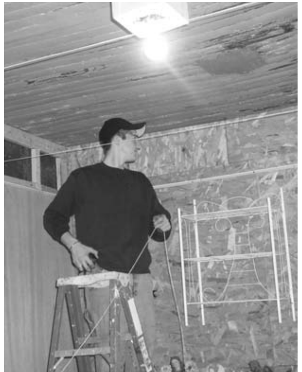
Max Markovich prepares to install a new ceiling.
